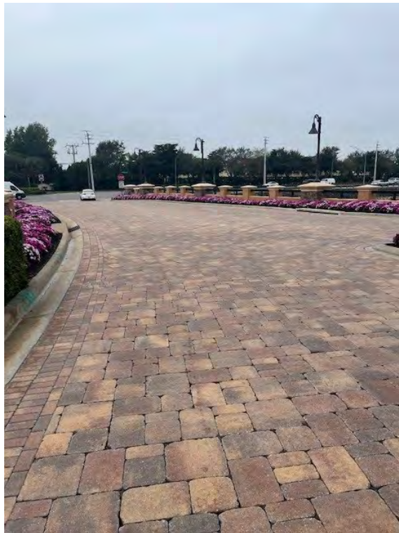
Entrance - Roadway & Lighting
