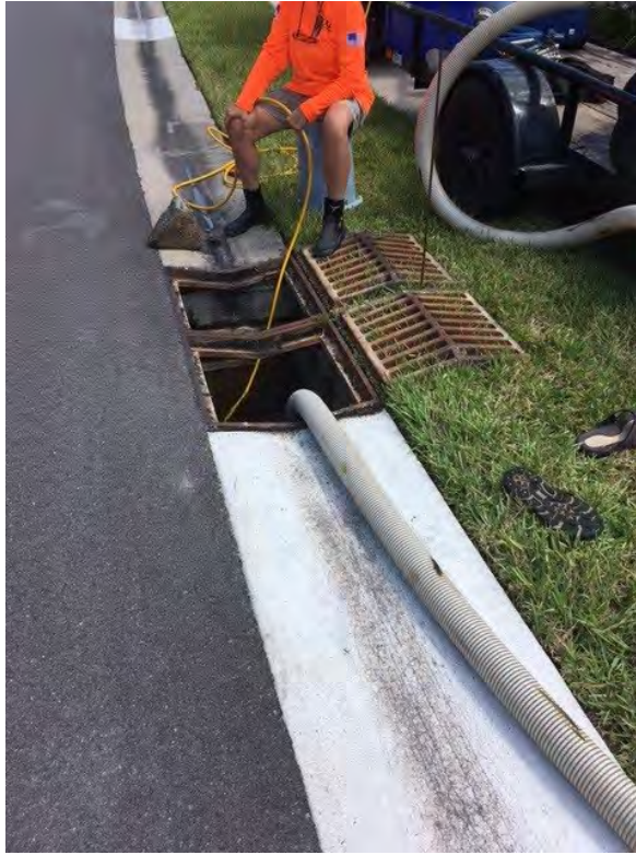
SWM - Drainage Structure
