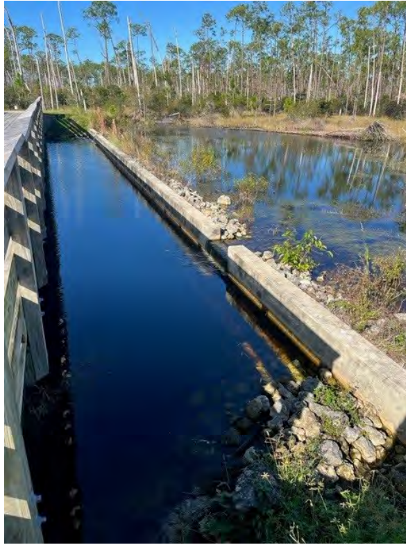
SWM - Flow Way Weir (North)
