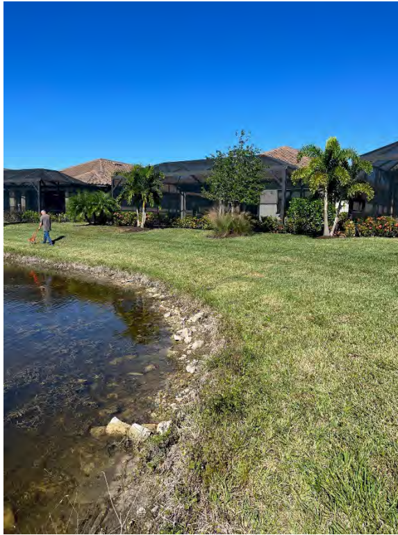
SWM - Lake Bank Slope
